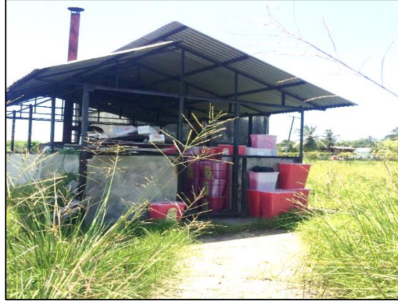
Fig.13 - Incinerator room West Demerara Regional Hospital Photo: Audit Office of Guyana
