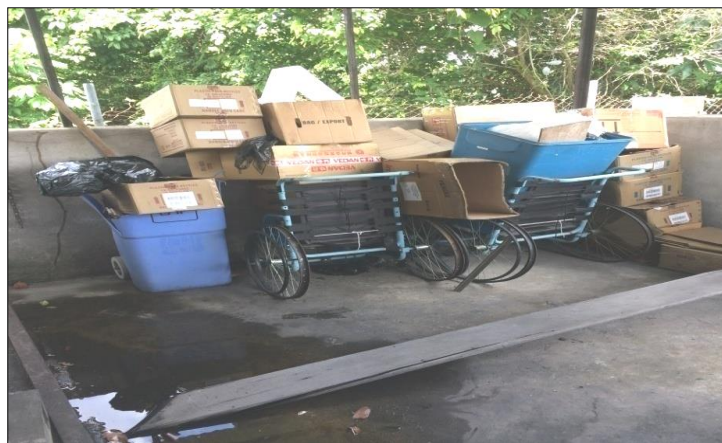
Fig. 14 – Unserviceable items in the incinerator room Linden Hospital Complex Photo: Audit Office of Guyana
